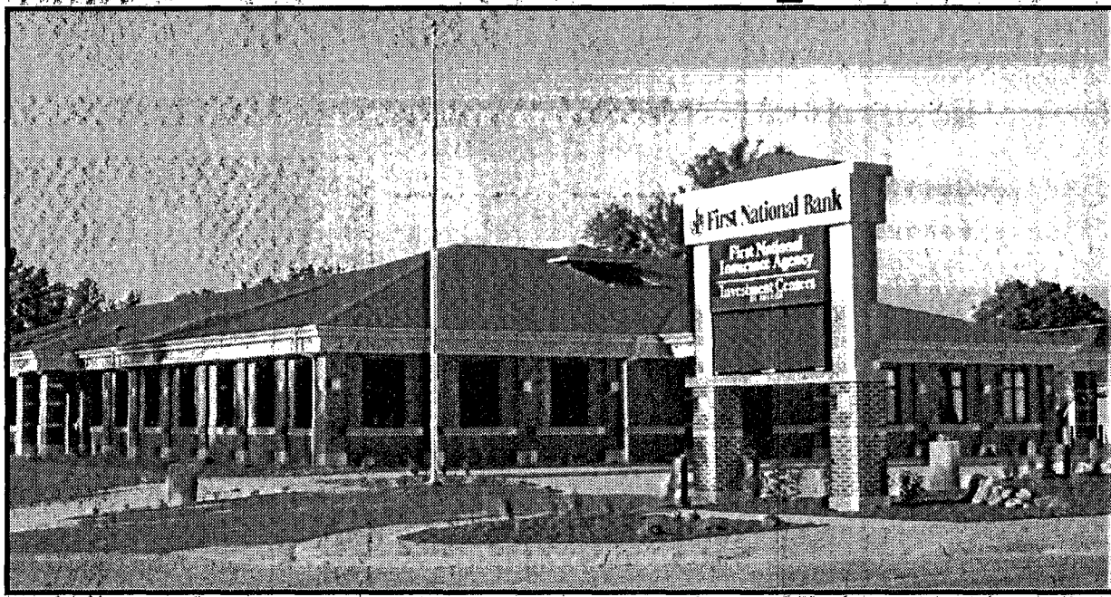
Nov. 13 is the targeted date for opening the doors for customer service at the new building of First National Bank of Wayne at 411 East Seventh Street.
